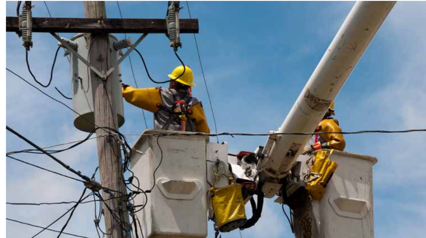
Workers attending to a power outage
