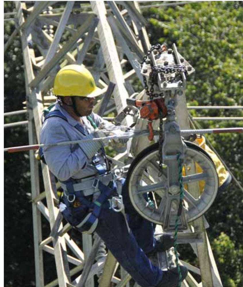
Optic Fibre line installation
