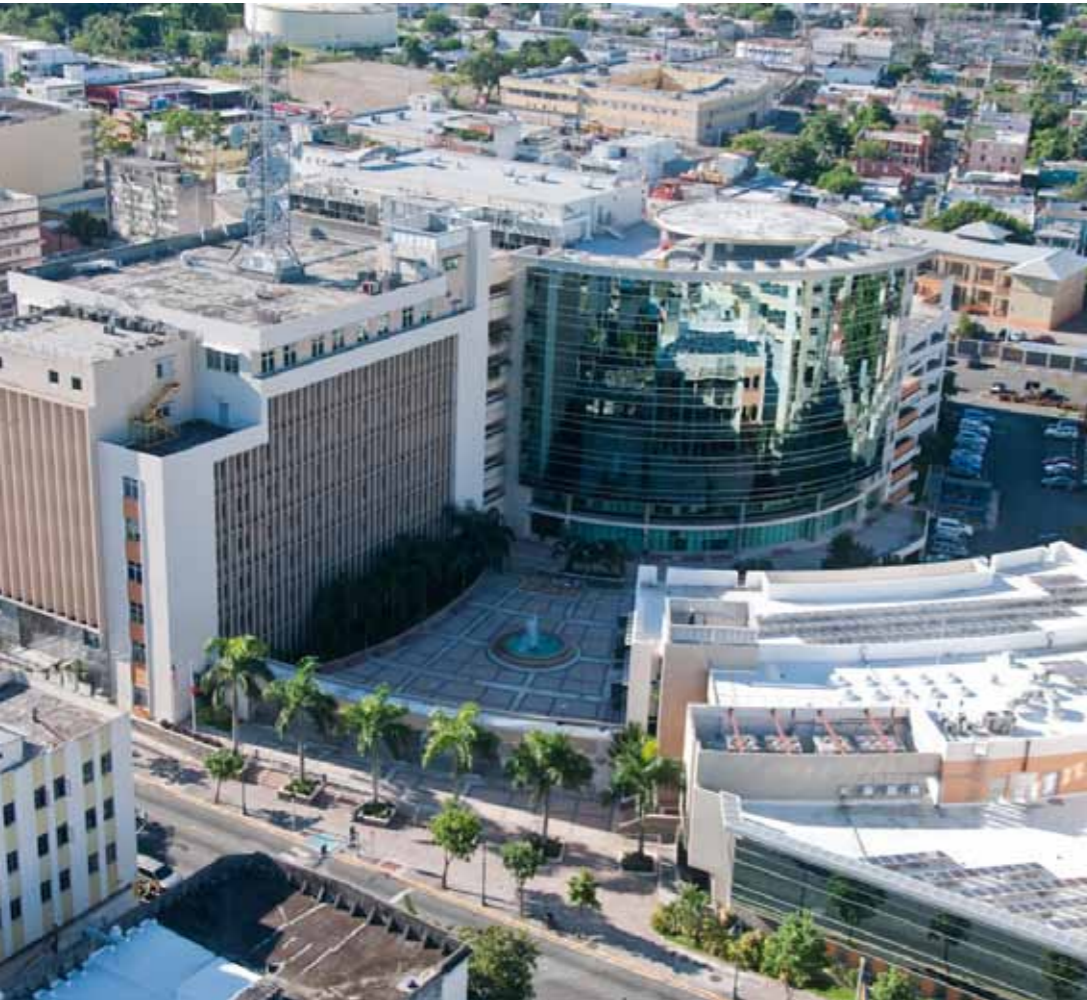
Puerto Rico Electric Power Authority Main Building
